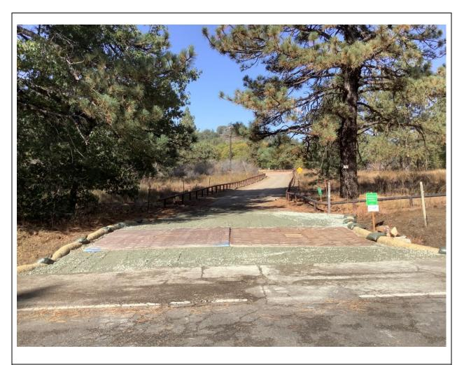
**Photo 5:** The entrance to Escondido Ravine Road (C 440) was stabilized with gravel and rattle plates to prevent trackout in accordance with the SWPPP.
