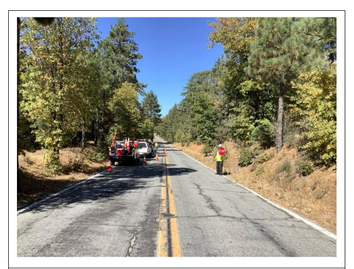
**Photo 6:** Cones, signage, and flagpersons were used to direct one-way traffic on Sunrise Highway during construction activities at Pole P40476 (C 440) in accordance with APM TRANS-02.
