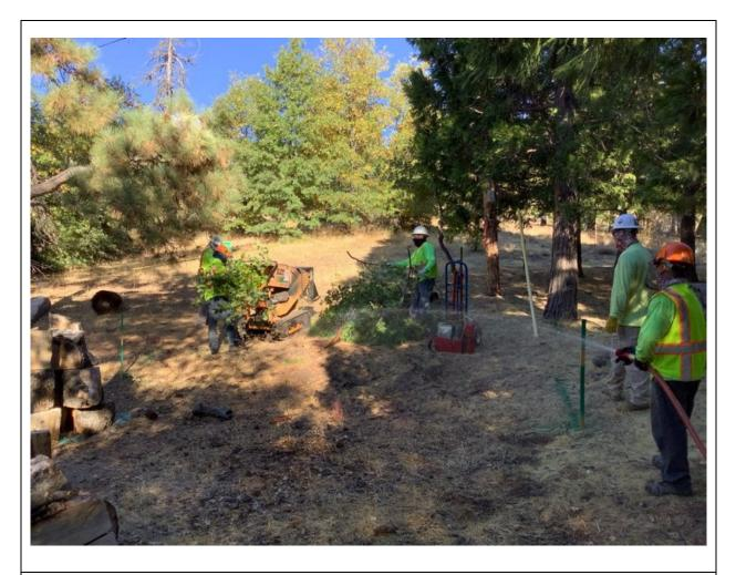
**Photo 4:** During chipping at Pole P40213 (C 440), a full set of fire tools was observed within 50 feet of the activity, at least 100 gallons of water with pump and hose were observed on site, and the area was wet down to prevent ignitions in accordance with the CFPPP for chipping on NFS land with a PAL D.
