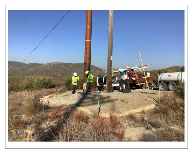
**Photo 2:** A crew was observed trenching for ground rod installation at Pole P198439 (C 79B) within clearly delineated work limits in accordance with MM BIO-1.
