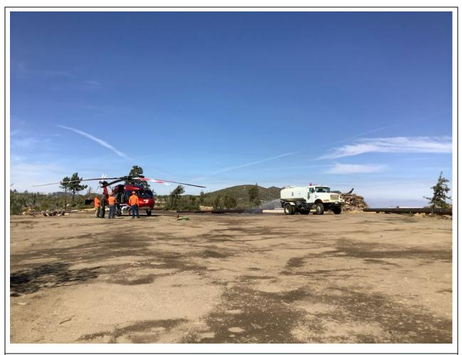
**Photo 1:** A water tender was observed applying water at Shrine Camp Staging Yard (C 440) prior to helicopter operations to minimize dust emissions from rotor wash in accordance with APM AIR-02 and the Aviation Safety Plan (MM PHS-5).
